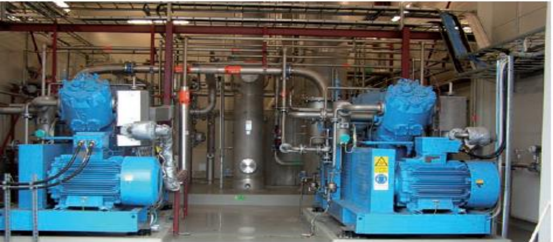
Photo 7. Kristianstad, Sweden, upgrading plant with a water scrubber. In the back the absorption column, flash tank and desorption column can be seen.
